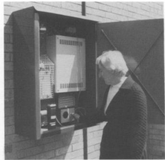
4. The scheme has been used to replace resident wardens in grouped housing schemes. The mobile warden checks the alarm outside the scheme to see which person to visit
